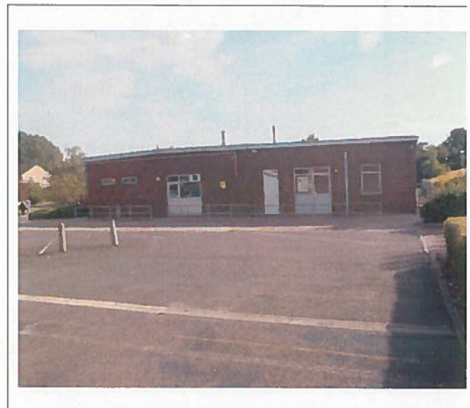
Car park – northern side
